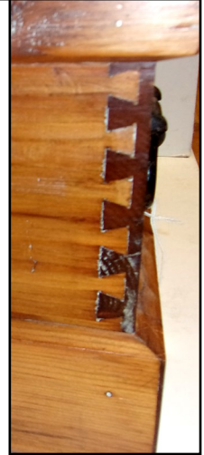
Chest with close up of corner showing dovetailed joints
